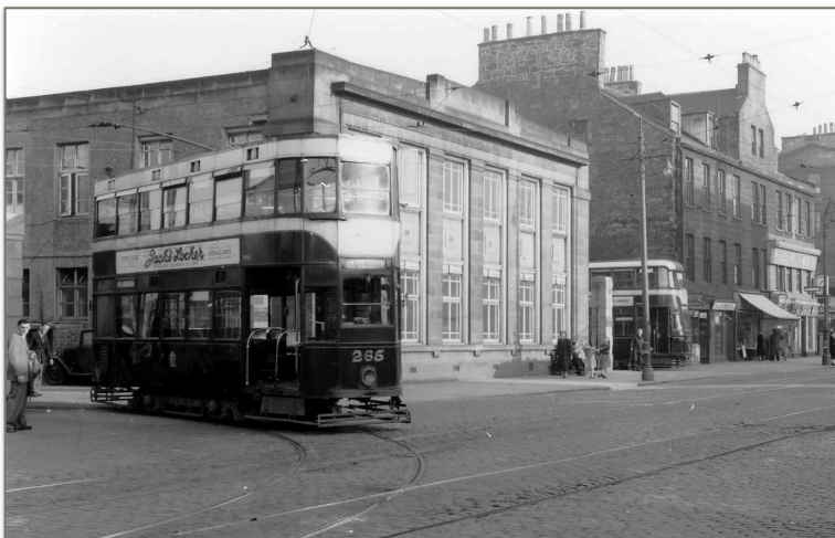
Pic 3: Car 265 exiting the northern entrance and able to go directly into service. This car was one of two all steel cars built by Metropolitan Cammel of Birmingham in 1933 which had the distinctive roof design similar to the 1932 experimental tram No. 180 built by Edinburgh Corporation at the Shrubill works. A streamliner is seen peeking out of the south depot entrance.
