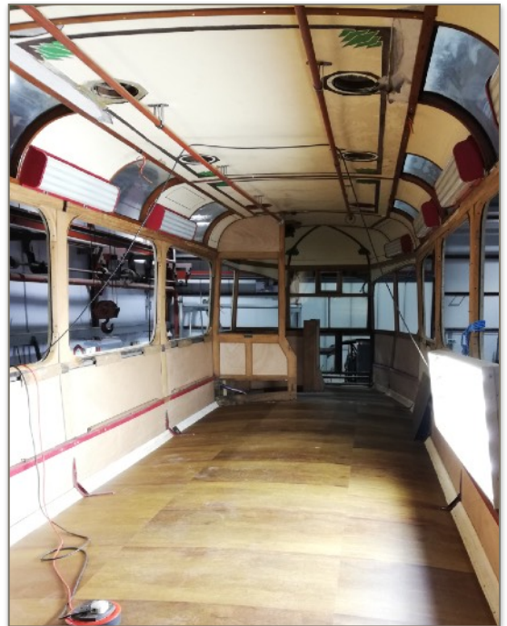
1245 Lights fitted and floors covered
